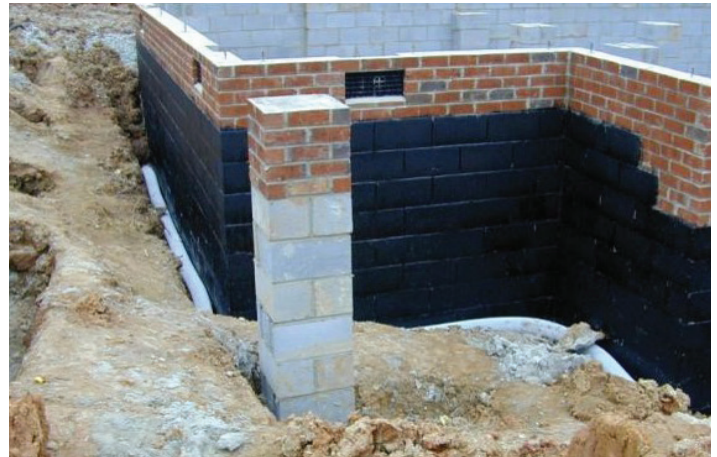
The below-grade concrete walls have damp-proof coating
