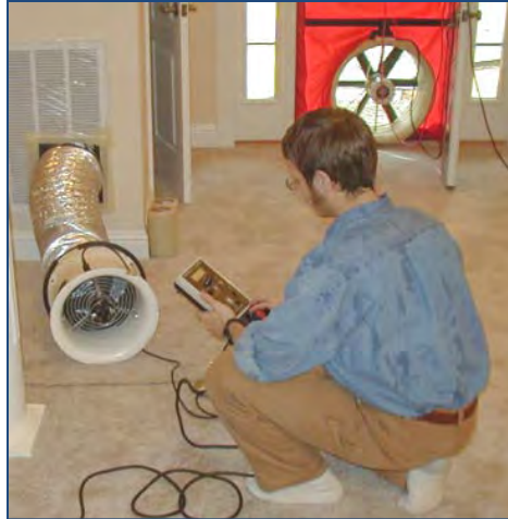
Figure 2. Duct pressurization test
