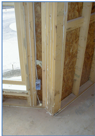
1. Complete all air sealing and rough-in work before installing insulation. Mask junction boxes.
