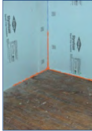
2. Install rigid foam and air seal.
